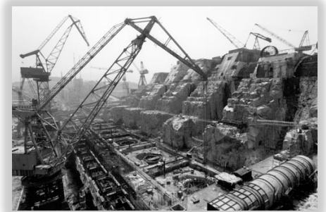
Construction Site of Three Gorges Dam
