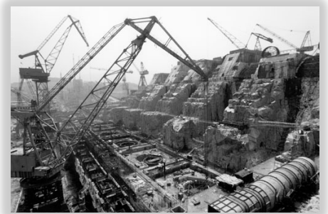
Construction Site of Three Gorges Dam
